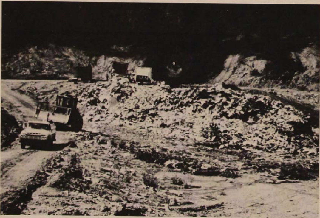
FIGURE 5. Heavy equipment used to cover landfill.
